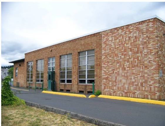
Main building (236A) south (side) elevation looking northwest.
