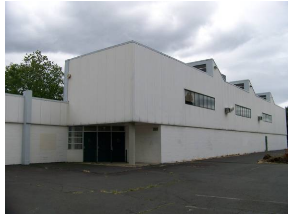
1975 Addition (236B), west (rear) elevation, looking southeast.
