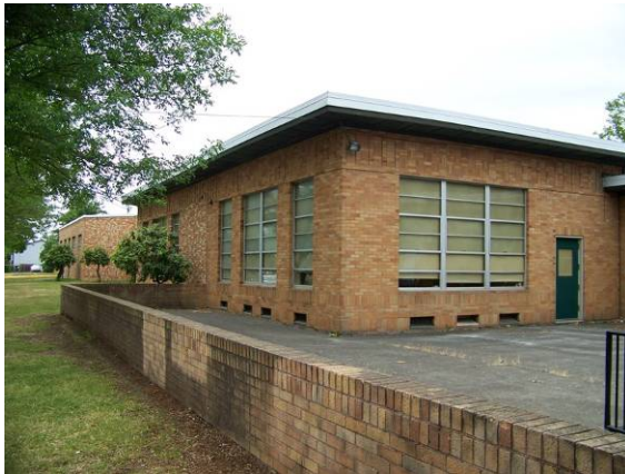
Main building (236A), east (front) elevation looking southwest.
