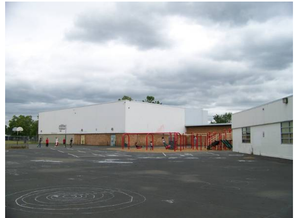
1975 Addition (236B) and Main building (236A), west (rear) elevations, looking northeast.
