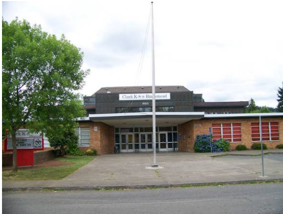
Main building (236A), east (front) elevation looking west.
