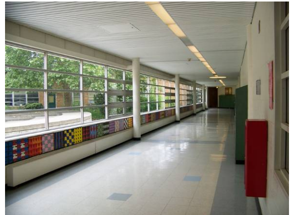
1975 Addition (236B), hallway between courtyard and wood shop/crafts room, looking southeast.
